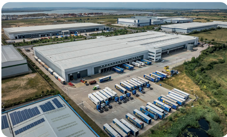
Transmec's customs warehouse at London Gateway is just minutes from the port. Image courtesy of Miru Visuals and DP World.
